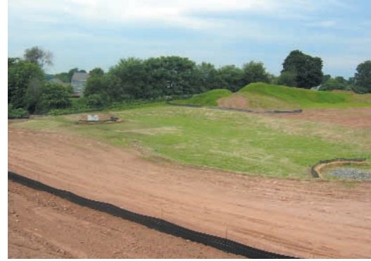
Sweeney graded two-acre retention pond without using a single grade stake.
